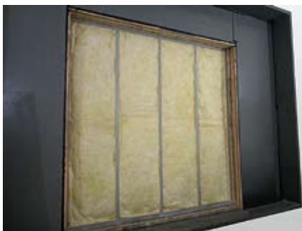
1 #1050R Self-Adhesive Tape, applied to the studs
