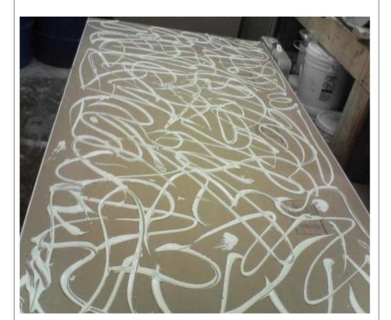
Figure 1: Typical Green Glue Application (photo by client)
